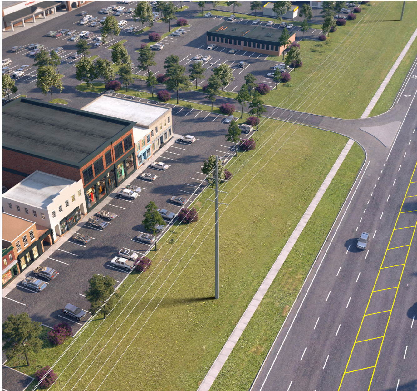
Steel Single-Pole Structure
