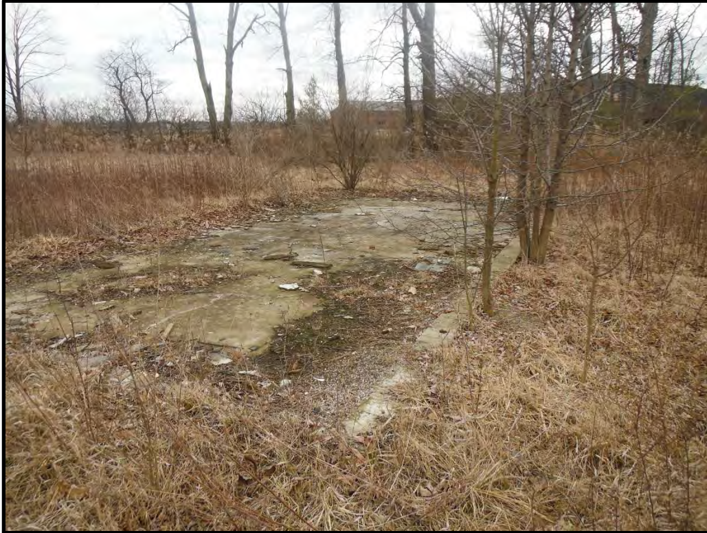
Figure 12. View of existing foundation.
