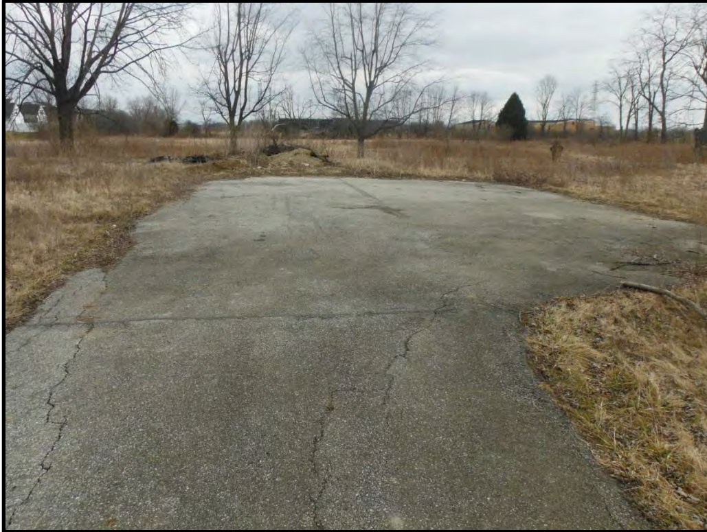
Figure 6. View of an existing drive within the project area.
