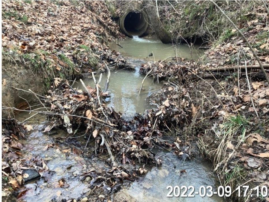
Photo Location 10. View of Stream 8 (intermittent). Photograph taken facing upstream, east.
