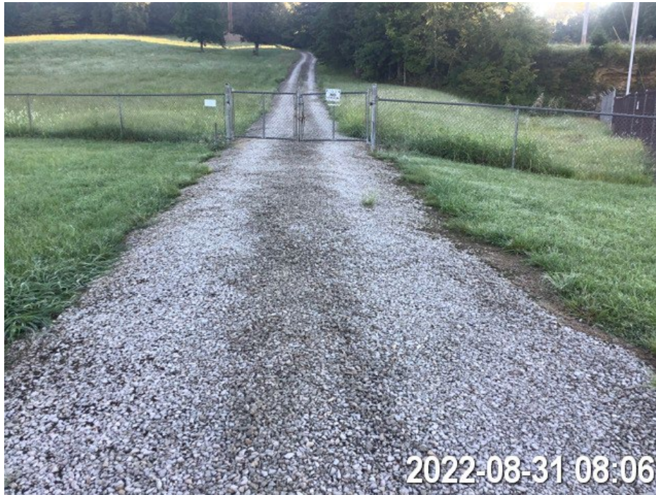
Photo Location 1A. View of gravel driveway in maintained lawn. Photograph taken facing north.
