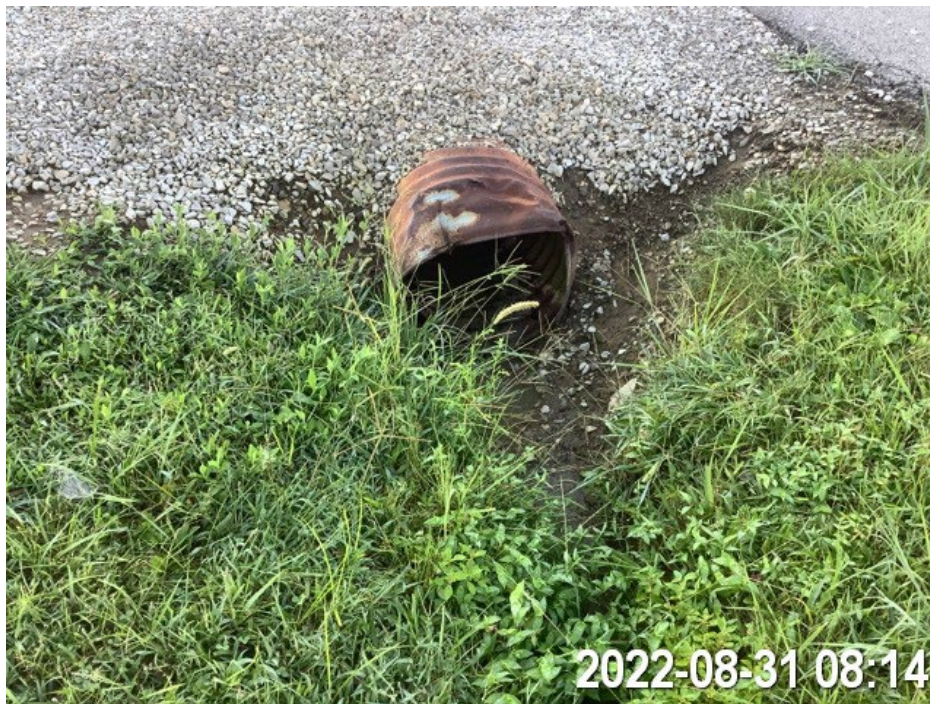
Photo Location 1B. View of typical culvert. Photograph taken facing south.
