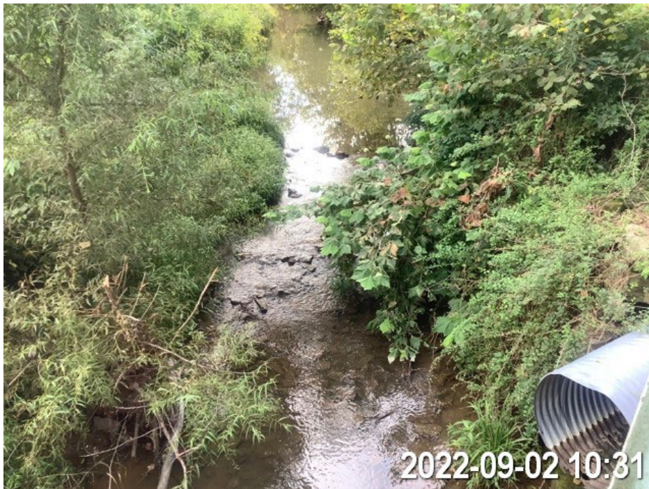
Photo Location 18A. View of Stream 13 (perennial; Lick Run). Photograph taken facing upstream, east.
