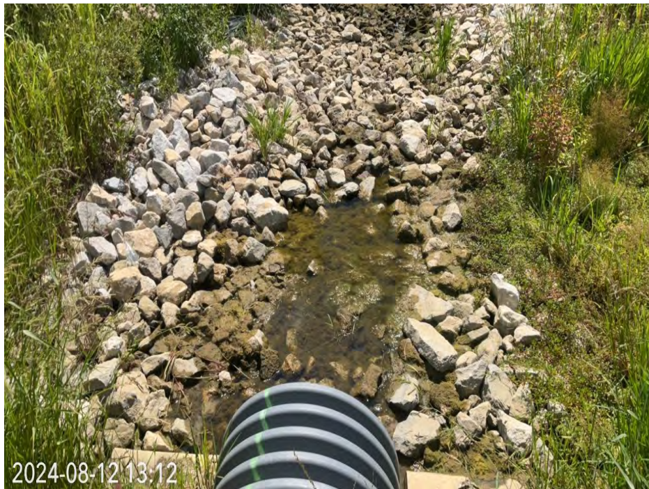
Photo Location 7. View of typical culvert. Photograph taken facing south.
