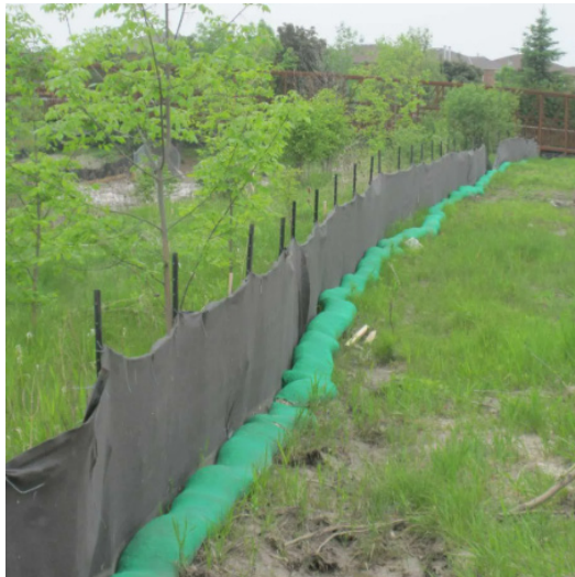
Example of Temporary Fencing to Control Sediment Movement
