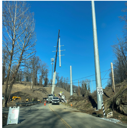
Example of Pole Assembly
