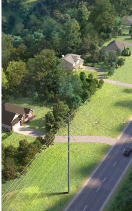
Typical Structure in Dierks
