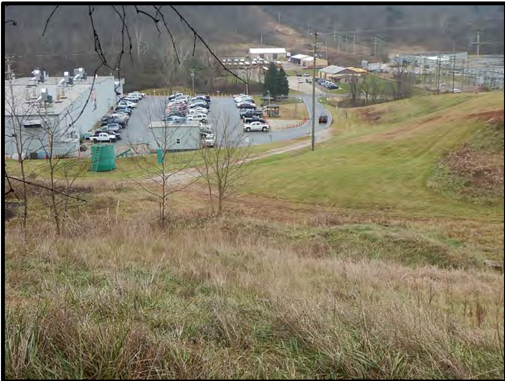
Figure 8. Typical sloped and disturbed conditions within the eastern access corridors.
