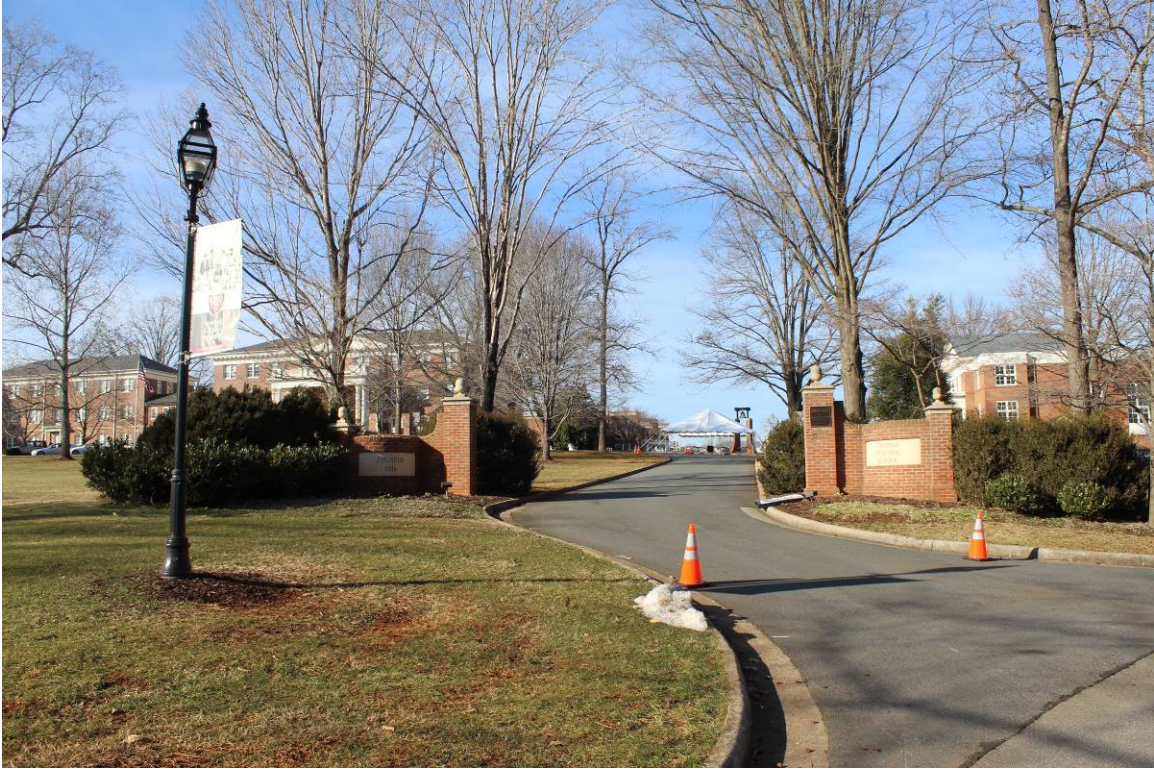
Photograph 5-28: Virginia Episcopal School campus entrance (Photo Location 1), facing north
