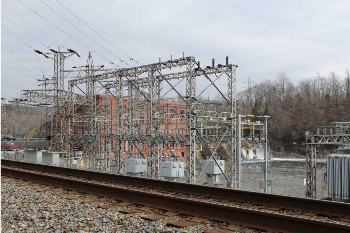
Photograph 5-39: Reusens Dam (Photo Location 1), facing northwest
