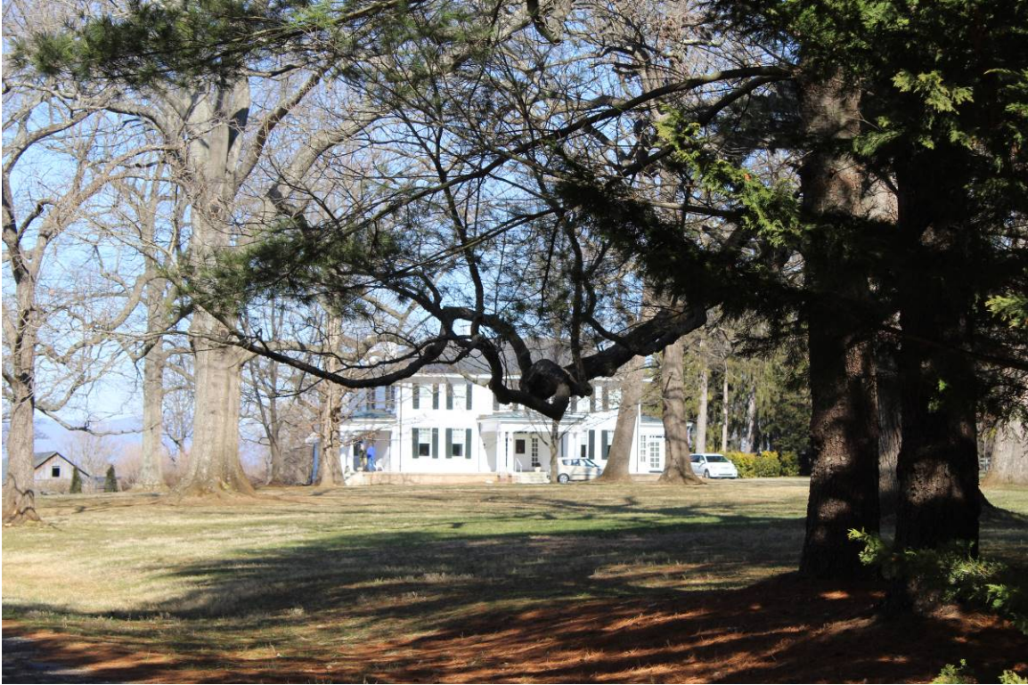
Photograph 5-13: Rothsay, front façade (Photo Location 1), facing north
