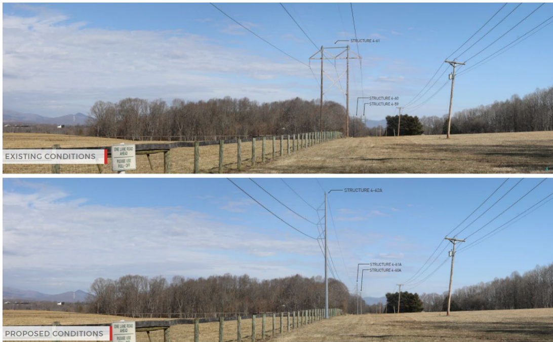
Figure 2. Comparable Existing and Proposed Single-Circuit Structure Existing Wood H-frame (top) and Proposed Steel Monopole (bottom)
