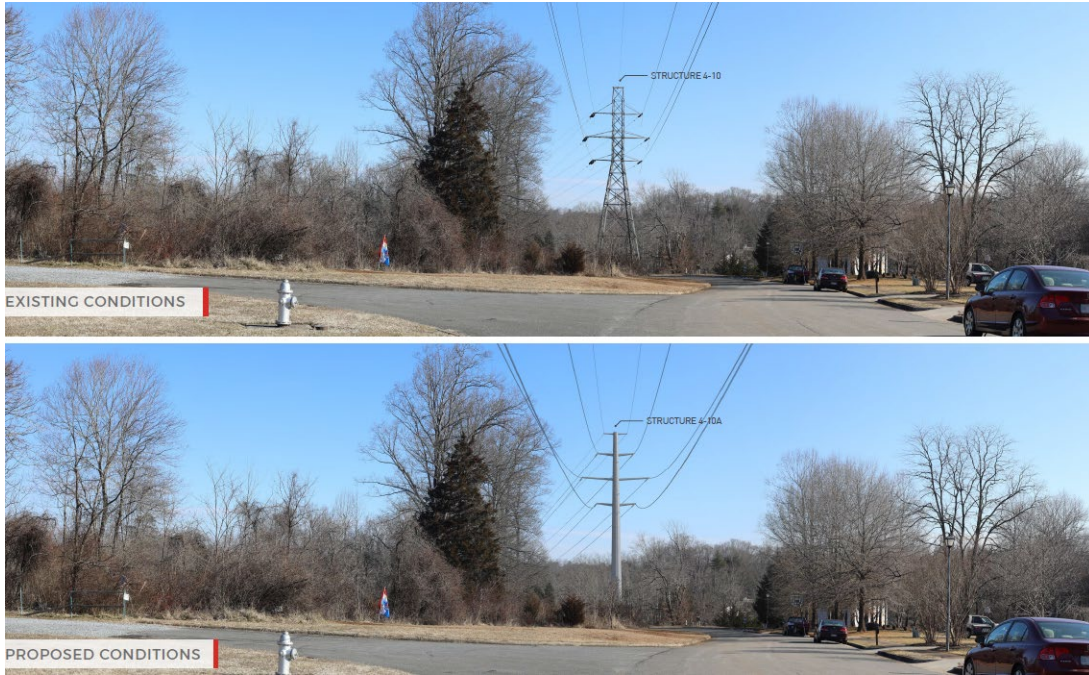
Figure 1. Comparable Existing and Proposed Double-Circuit Structure Existing Steel Lattice (top) and Proposed Steel Monopole (bottom)
