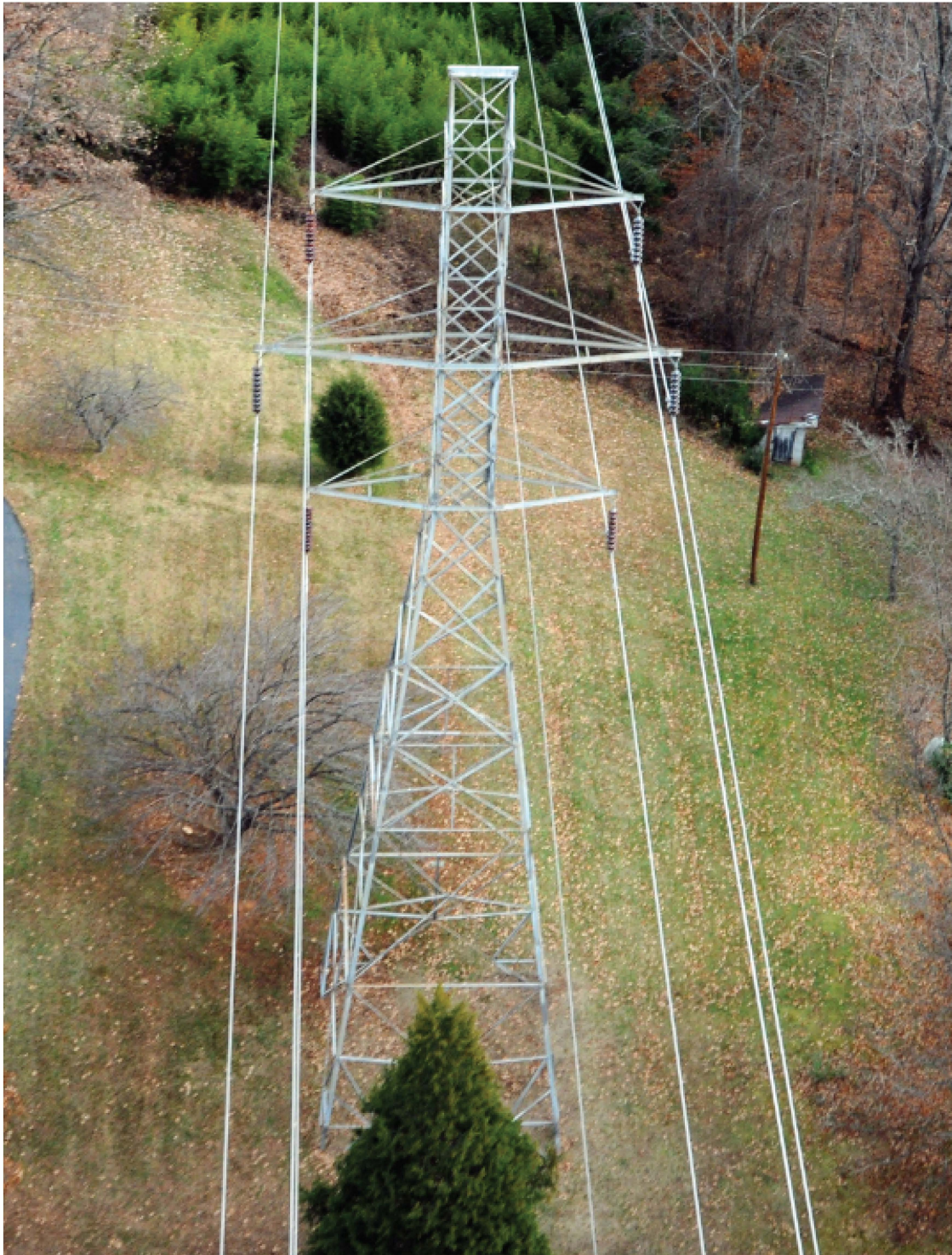
COMPARABLE EXISTING STRUCTURE PHOTOGRAPH
