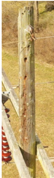
Figure 11 Structure 33: Pole Cavities
