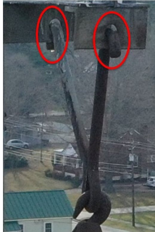
Figure 6 Structure 11: Structure Attachment Points and Corrosion of Insulator Hardware
