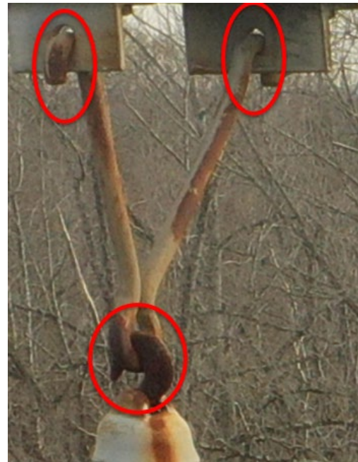
Figure 6 Structure 11: Structure Attachment Points and Corrosion of Insulator Hardware
