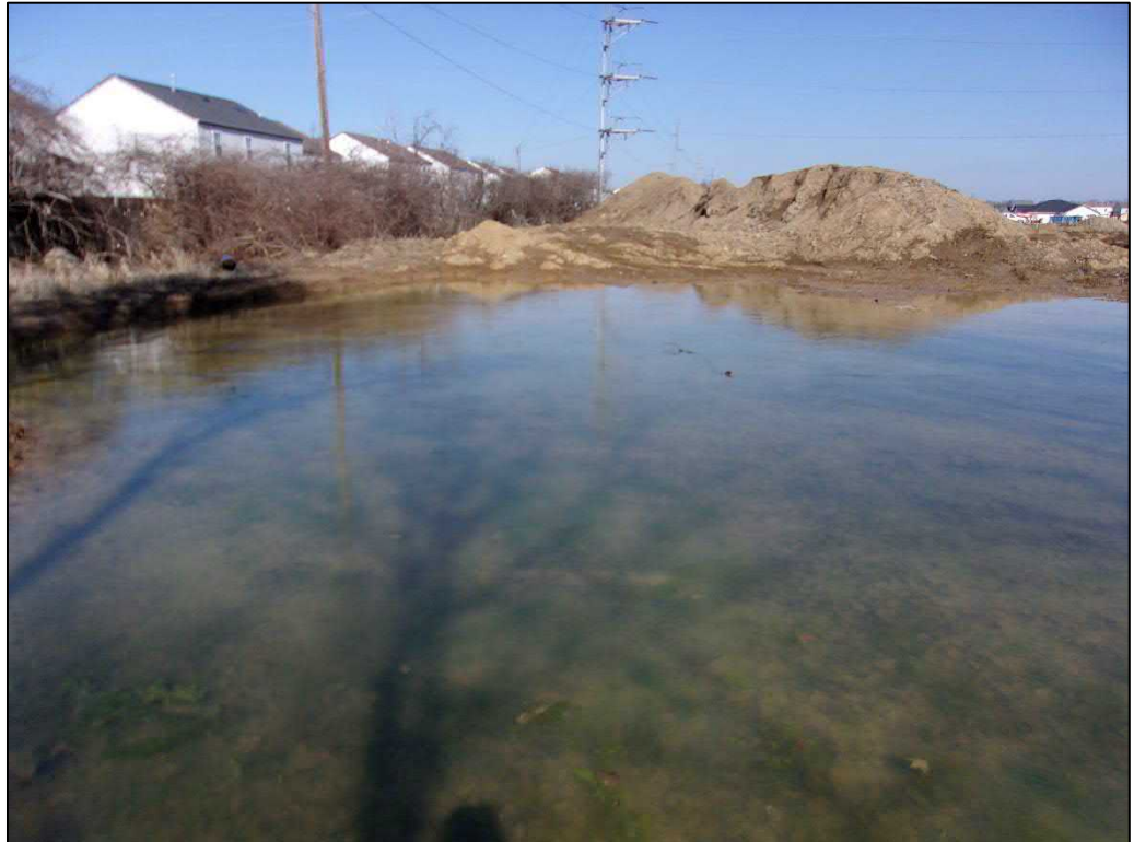
Detention Basin AS-2 facing north on February 19, 2020.
