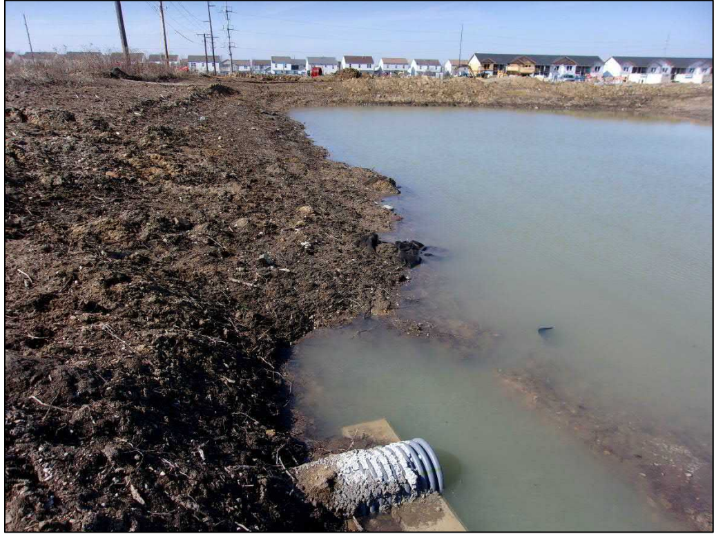
Detention Basin AS-3 facing west on February 19, 2020.
