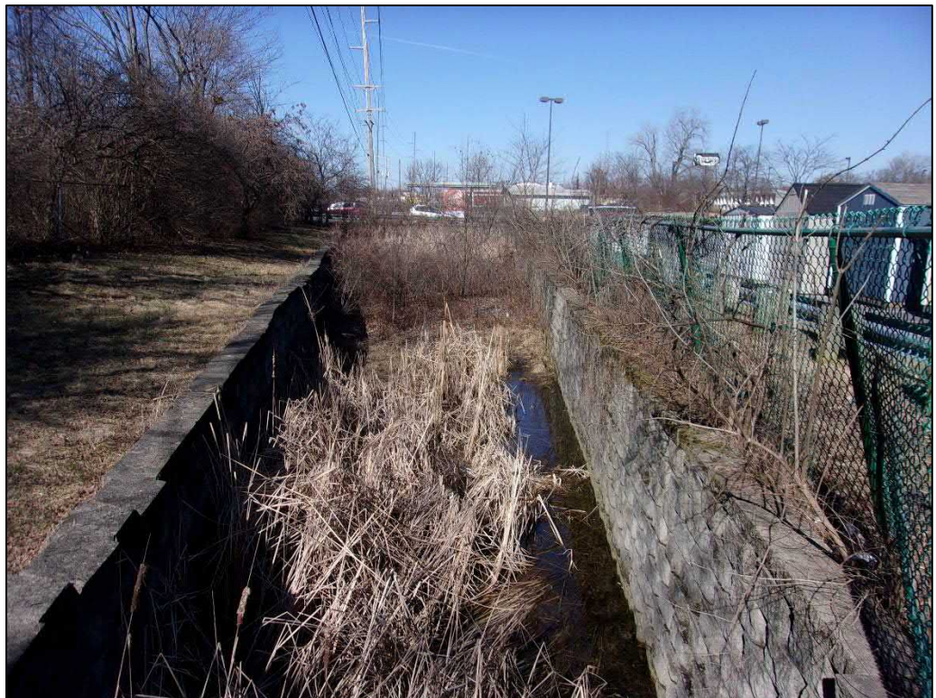
Detention Basin AS-7 facing north on February 19, 2020.
