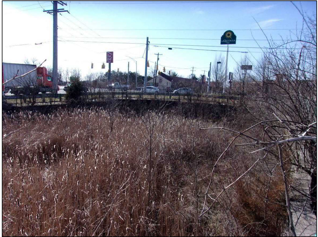
Detention Basin AS-6 facing west on February 19, 2020.
