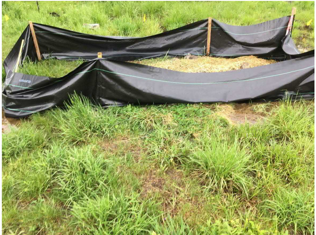
Wetland AS-4 (PEM), facing east on May 5, 2020.
